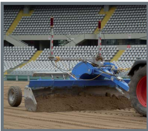
» Stadio delle Alpi – MOBA Dual-Laser-matic used for leveling works in the soccer stadium of AC Turin (Italy)
